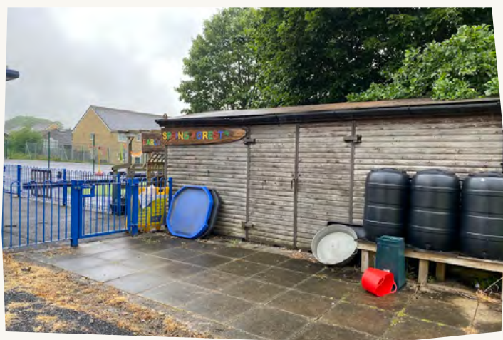
Shed before green roof
